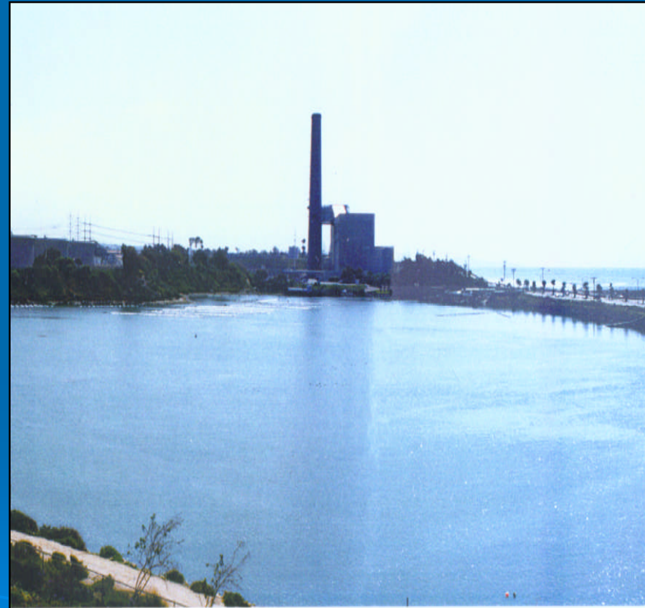
Encina Power Plant in Carlsbad, California
