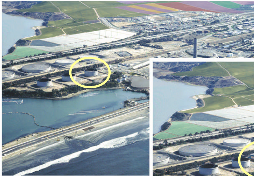
EXISTING SITE CONDITIONS
